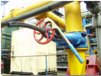
Photo 7 and photo 8: The key facilitates evidently the maneuver of the horizontal and vertical valves.
