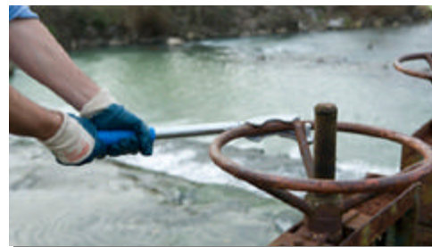
Photo 7 and photo 8: The key facilitates evidently the maneuver of the horizontal and vertical valves.
